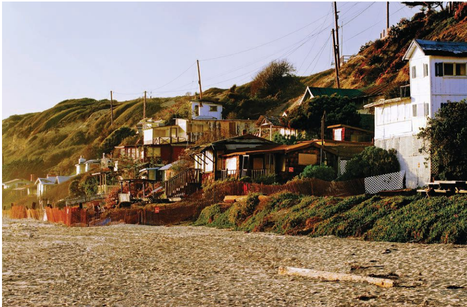
Seventeen cottages await restoration on the North Beach.
